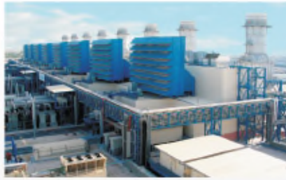
Az Zour Power Plant, Kuwait
